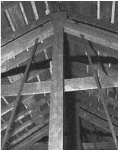
Iron rods support scarfed tie beam.
