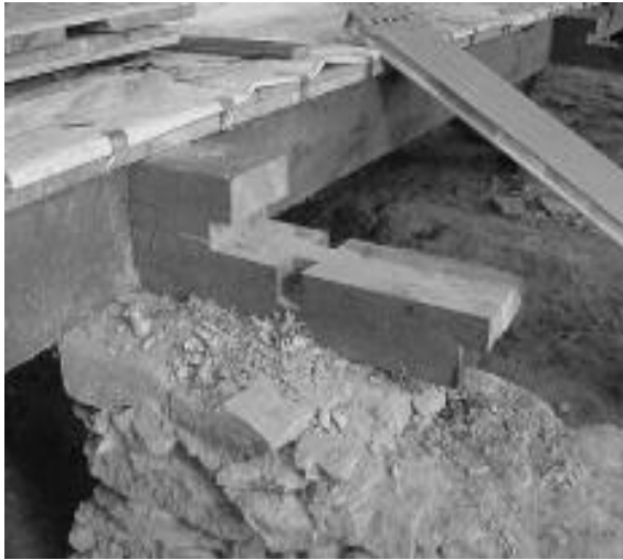
Edge-halved scarf in floor girder. Notch carries joist.
