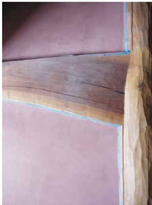
Timber frames and clay walls. Top right, Tom Basler applies water in preparation for the second coat of plaster.
